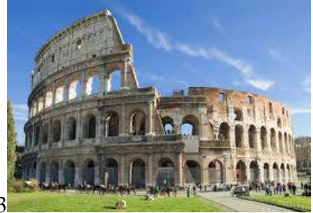
3 needs some pointing
